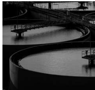
Water Treatment Center
