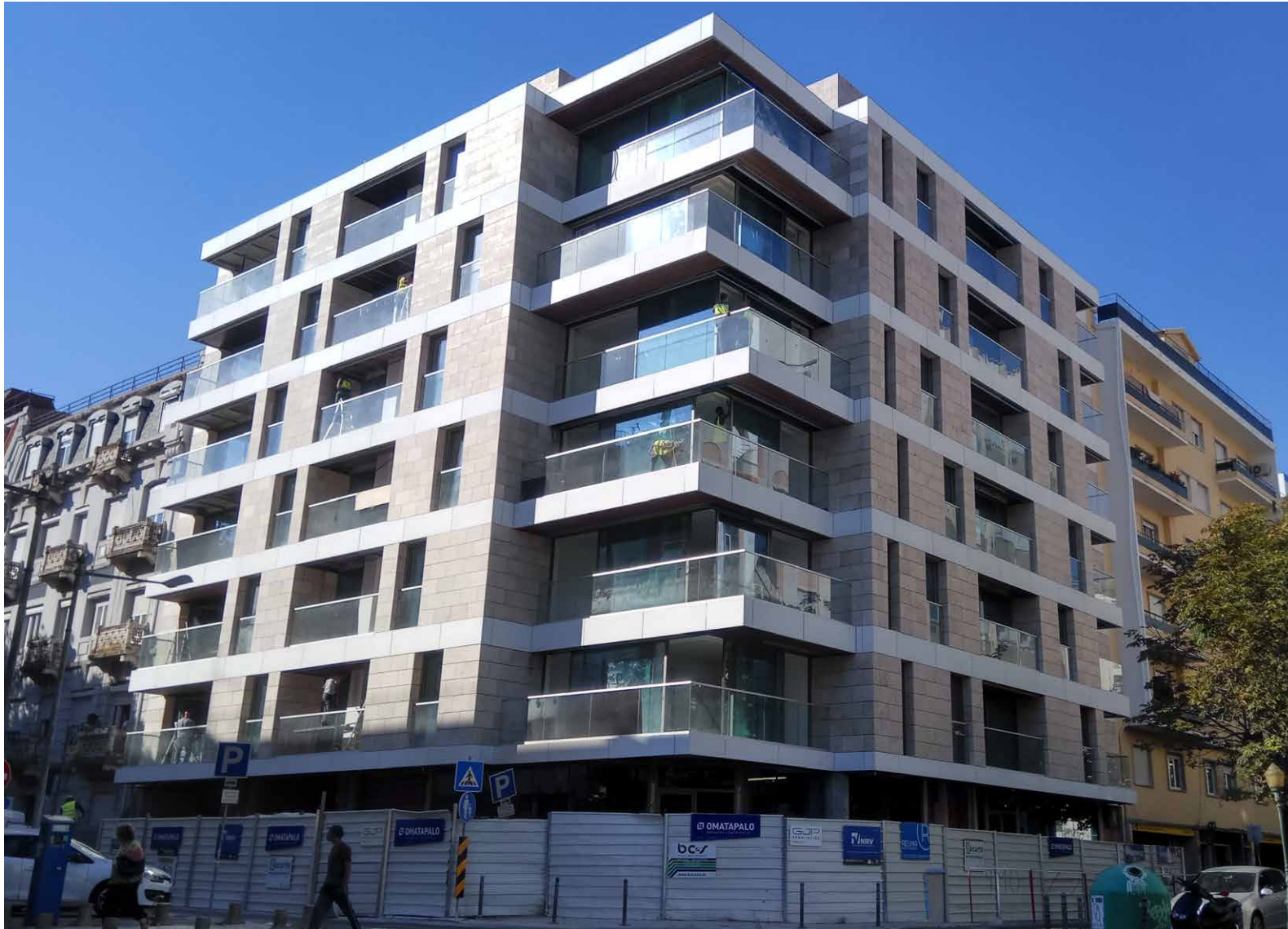
Work in Progress. Residential building in Rua de Pinheiro Chagas, Lisboa.
