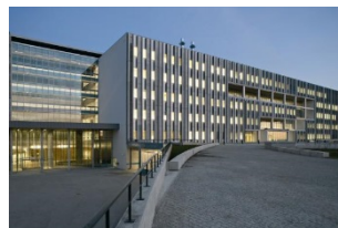
Novo Hospital de Braga
